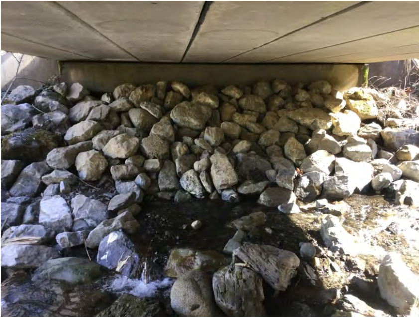
Right Bank Abutment when facing downstream
