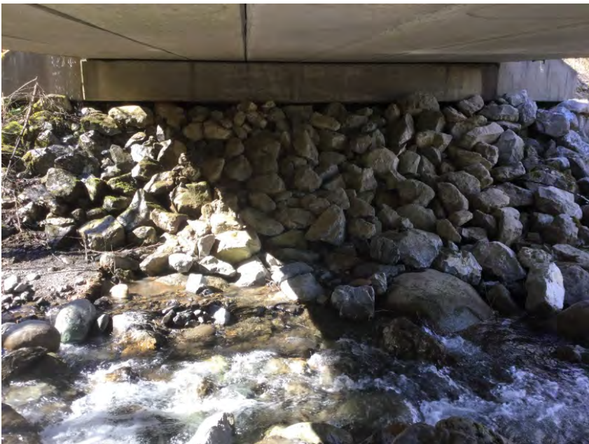
Left Bank Abutment when facing downstream
